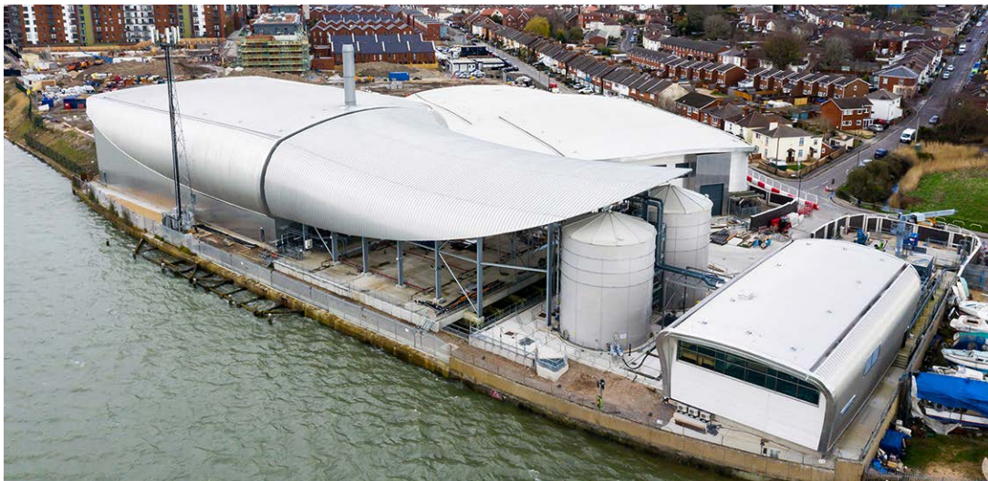
Woolston Wastewater Treatment Works was built to be resilient to future threats from flooding
