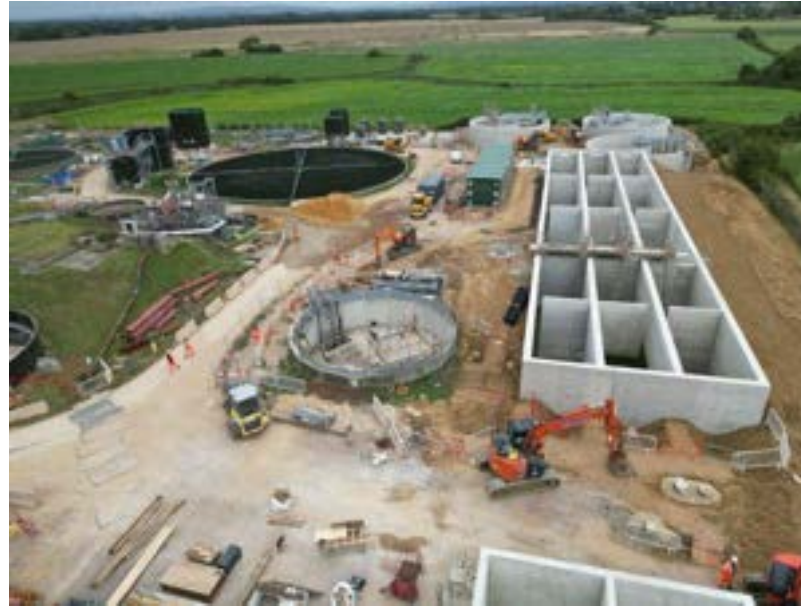
Pagham Construction of new installations
