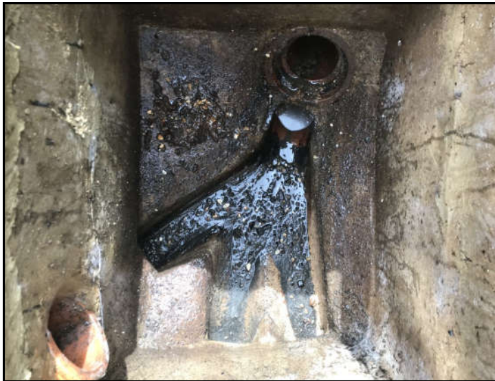
IC1 - CLEARED AT TIME OF SURVEY
